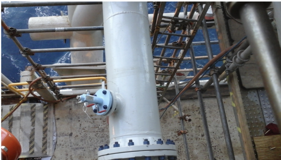
Figure 2: Installed sample probe for a sampling system
