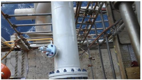
Figure 2: Installed sample probe for a sampling system
