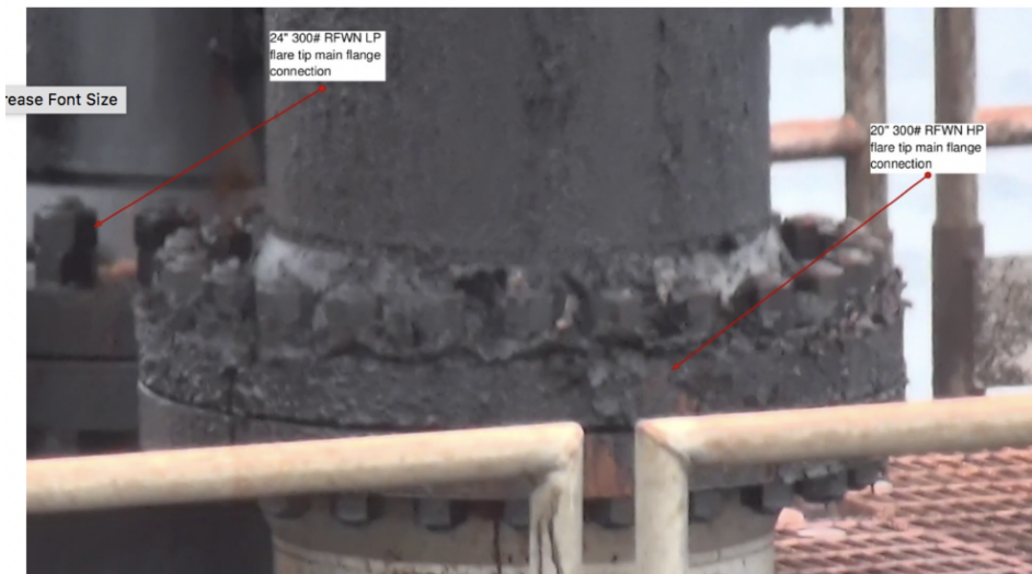
Figure 4 - Flare Tip Flanges
