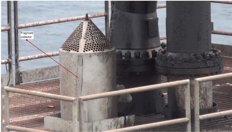
Figure 5 - Ballistic Ignition System Catcher
