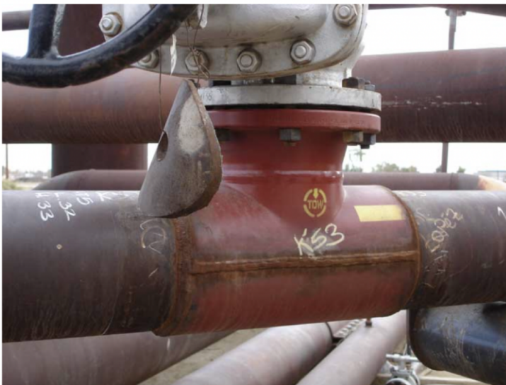
Figure 3: Completed hot tap with removed coupon
