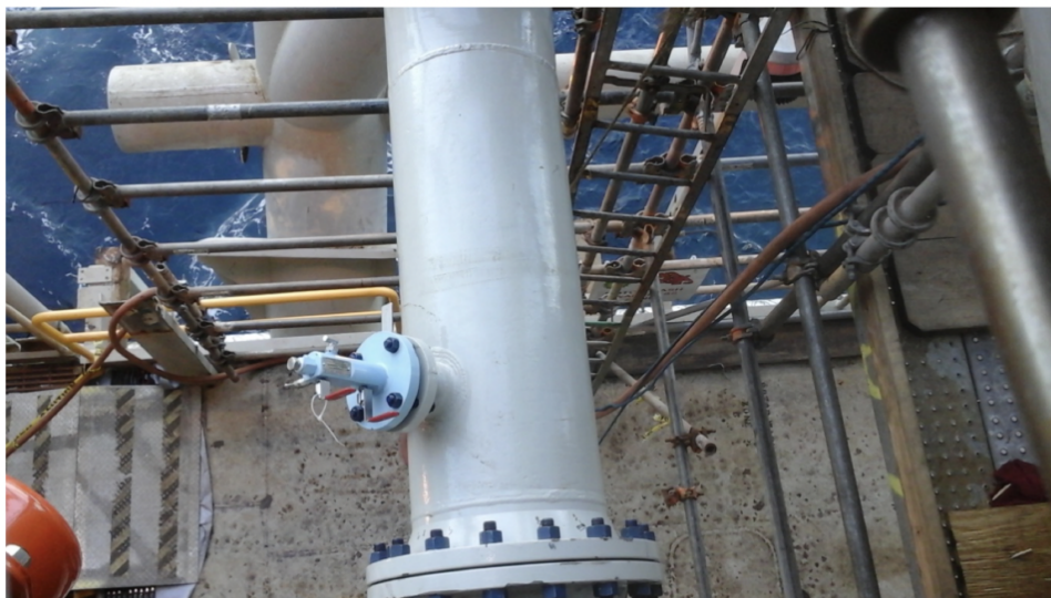
Figure 2: Installed sample probe for a sampling system
