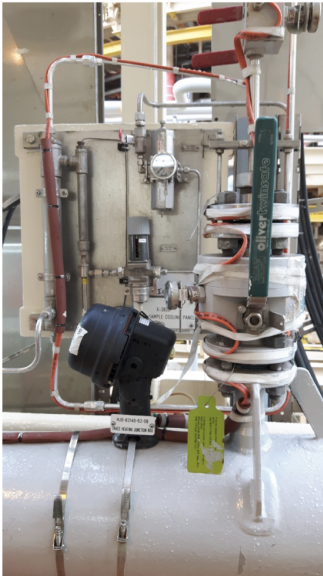
Figure 2: Installed retractable sample probe for a sampling system
