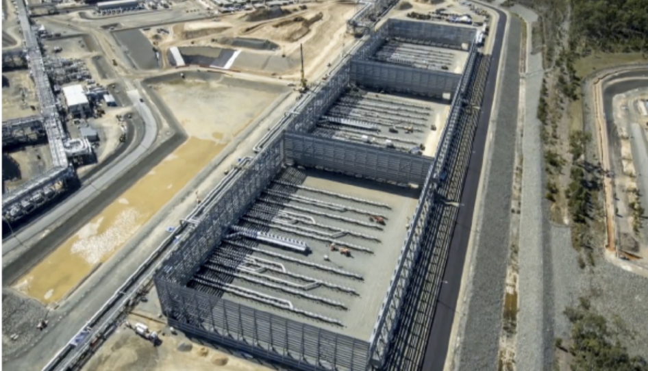
Figure 1: Example of multi-point ground flares installed for LNG service
