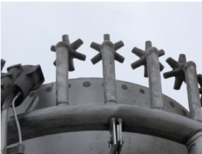
Figure 2: Steam-assisted flare tip with upper ring steam injectors
